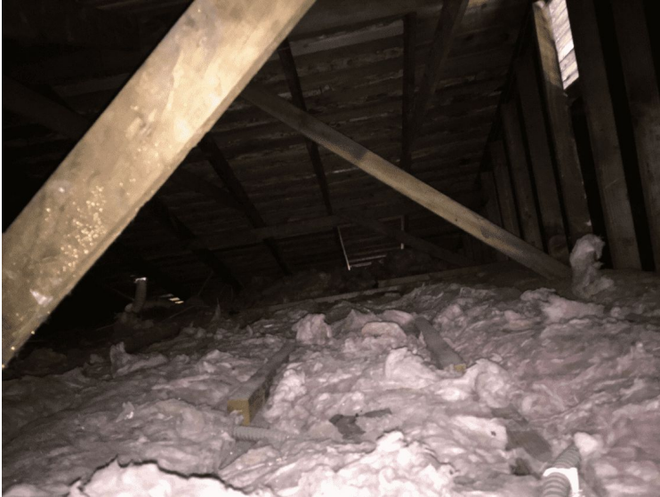
Today: Attic, some insulation Recommend: R-38
